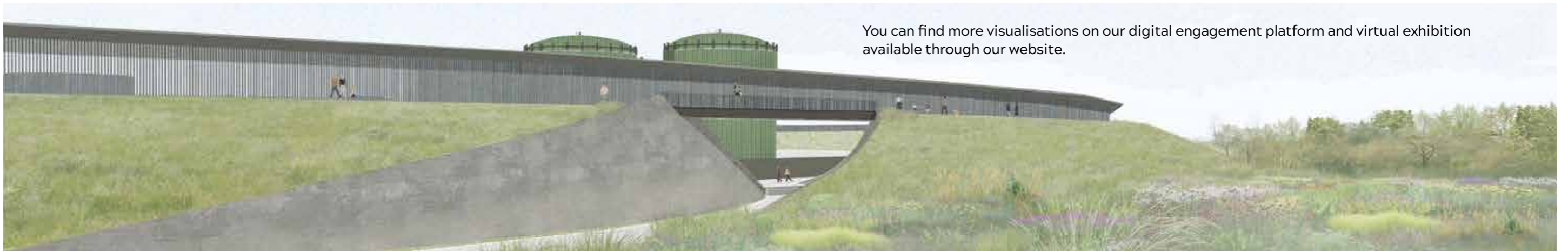
Illustrative visualisation of the anaerobic digester cladding with a natural, matt finish behind additional screening on top of the earthwork bank
